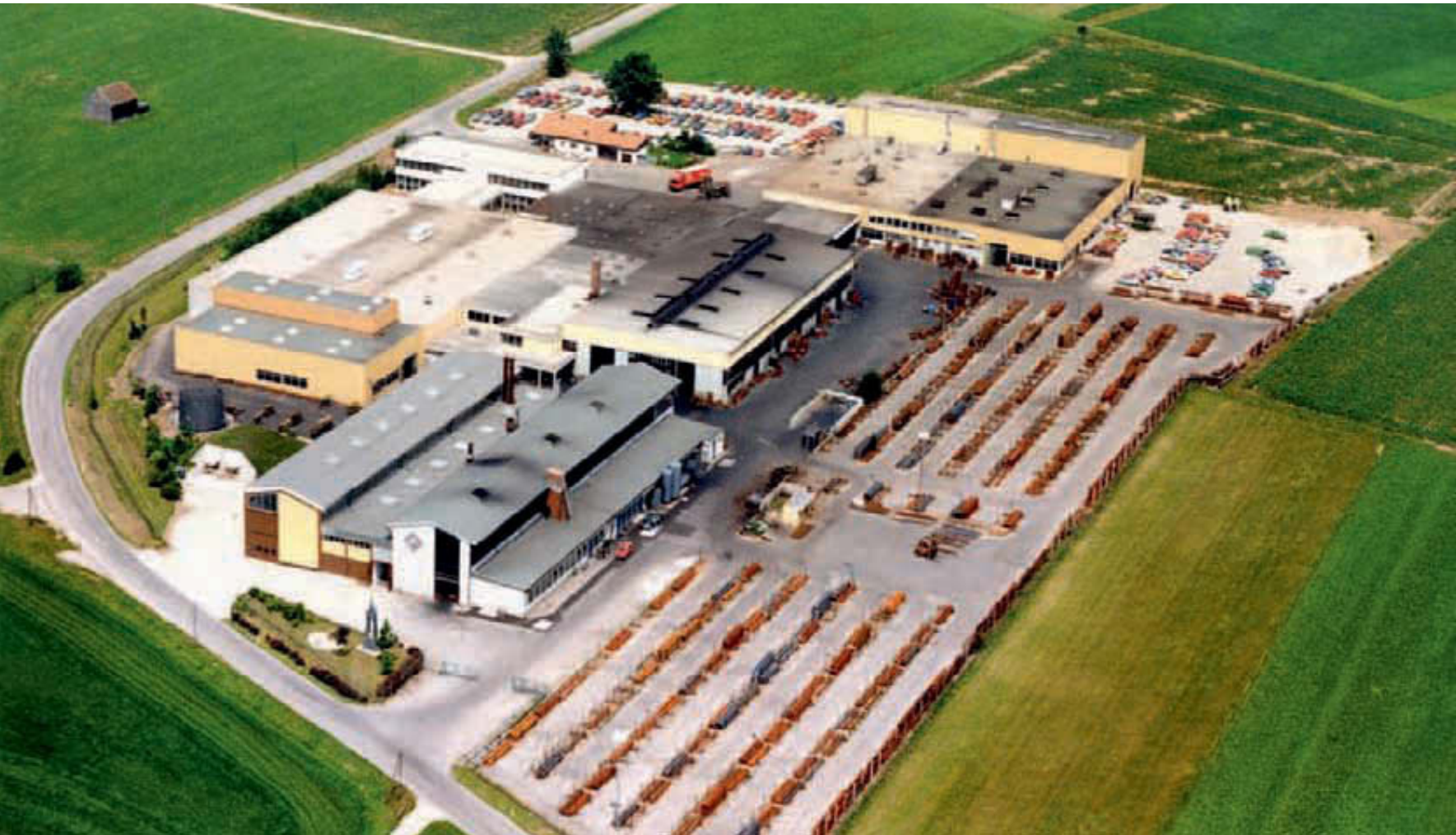
The main plant in 1985
