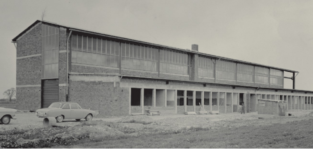
Hall 1 under construction in 1962
